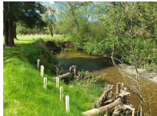
Bank Stabilization Project Completed Through NRSP
