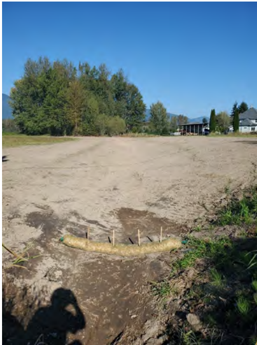
2020 DU project to reestablish historical drainage flow path in Sedro-Woolley.
